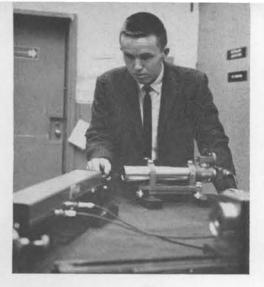
LASERS occupy the interest of Jeff Edixon (8151-1), who is completing his last period in the co-op work-study program at Livermore Laboratory. The laser is being developed for use as an interferometer, a sensitive measuring instrument.
